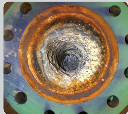
Spool pulled downstream from scavenger injection site before treating
